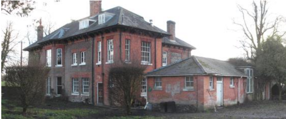
Sharcott Manor (from the rear/ side) and outbuilding to be demolished (2019 photo)
